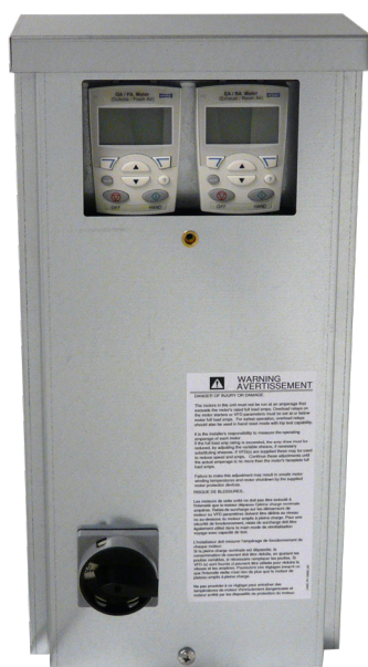
FIGURE 14.6.1 VFD KEYPADS IN EBOX
