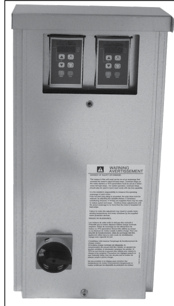
FIGURE 14.6.5 VFD KEYPADS IN EBOX
