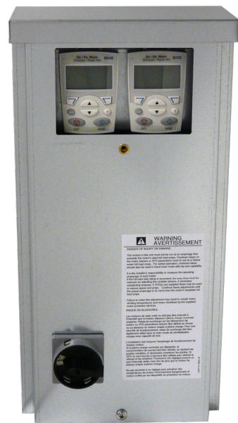
FIGURE 15.6.1 VFD KEYPADS IN EBOX
